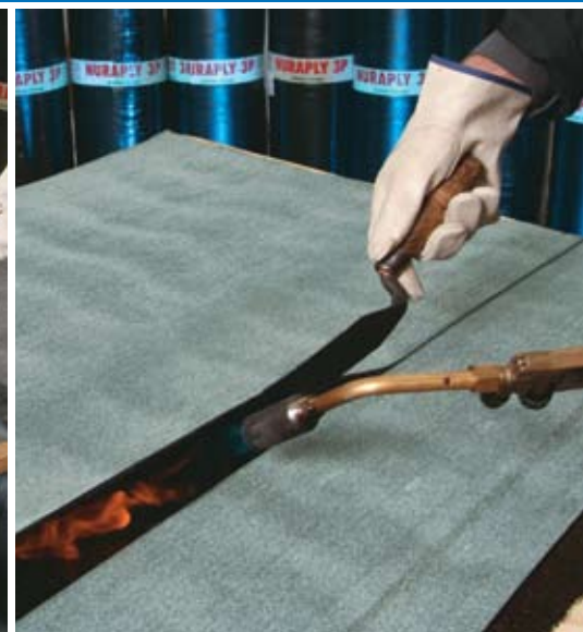
C/ Welding lap joints
