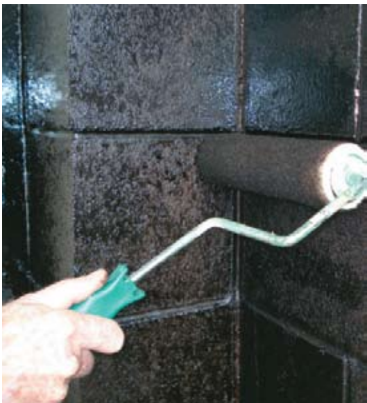
A – Nuraflux primer applied to substrate
