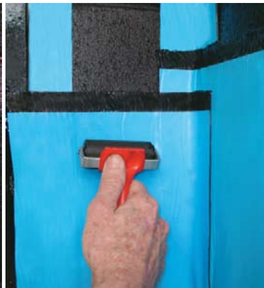
C – Roller used to ensure good seal
