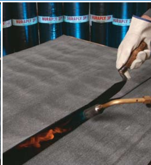
B/ Welding lap joints
